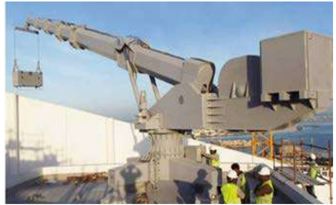
Roof machine with Standard Cradle
