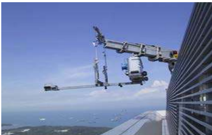
Telescopic Jib with Telescopic Cradle
