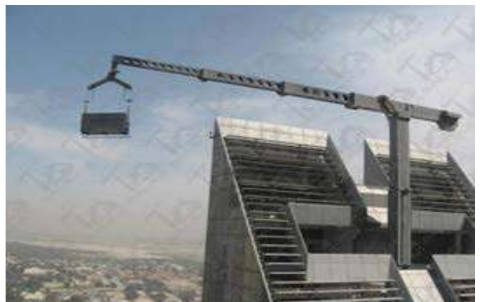
Telescopic Jib with Telescopic Mast
