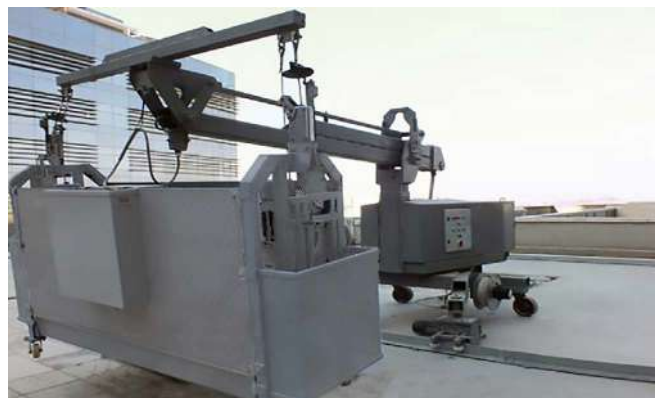
Roof Machine on Guide angle
