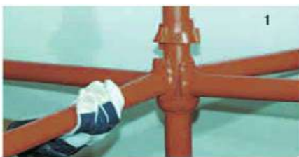
Fix ledger blade ends into lower cup
