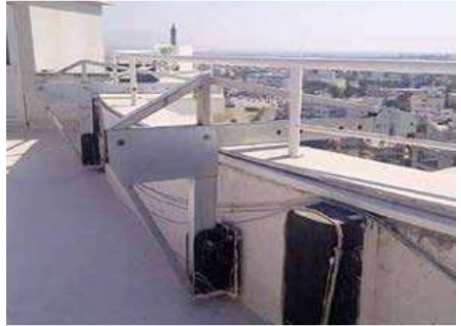
Parapet Mounted Low Rise Davit
