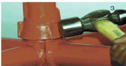
Rotate the top cup with hammer to lock the blade ends
