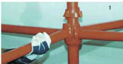
1 Fix ledger blade ends into lower cup
