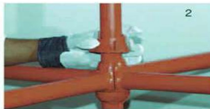
2 Position the upper cup over the top end of ledger blades
