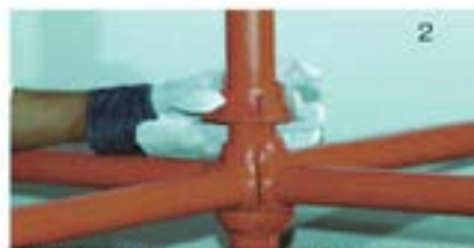
Position the upper cup over the top end of ledger blades
