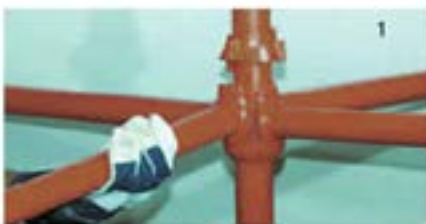
Fix ledger blade ends into lower cup
